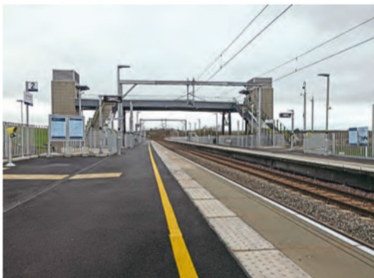
The new station at East Linton, which was due to welcome passengers from December 13. Network Rail.
