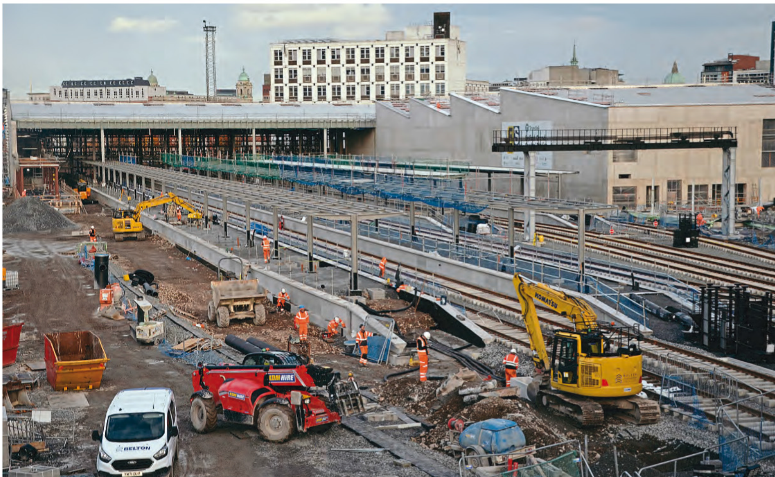
Track and platforms in the process of being completed at Belfast Grand Central Station on November 8. This will be the new transport hub in the city and will result in the closure of the current Great Victoria Street Europa bus and rail station. The new hub will feature eight platforms, 26 bus stands, increased cycle and taxi provision, track and signalling improvements, car parking and a new public square, and is due to open in late 2024. Chris Playfair.
