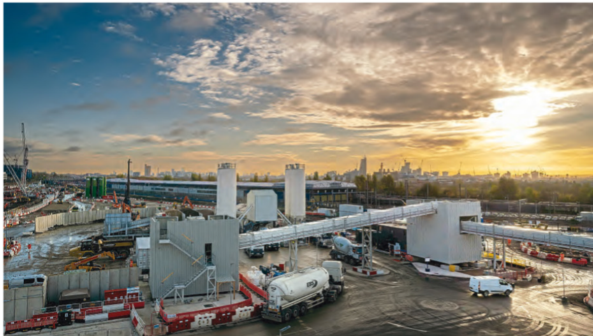
Initially HS2 trains will terminate at Old Oak Common, with connections into London available via the Elizabeth Line. This is a view of the site looking towards the Great Western Main Line and Hitachi's North Pole depot. HS2 Ltd.
