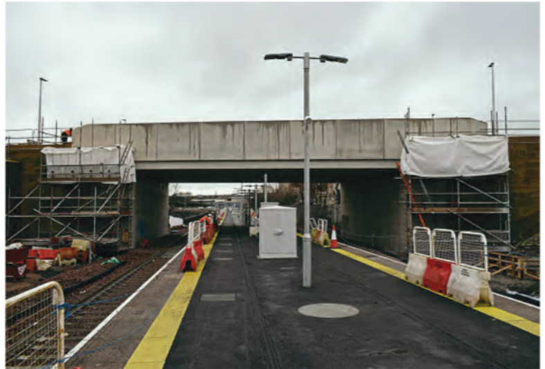
Leven station on December 15, 2023. The circular cover in front of the light is for the electrification stanchion. Although wires are not being erected ahead of the line's reopening, piling has been undertaken so this work can be undertaken quickly when wiring is authorised. Richard Clinnick
