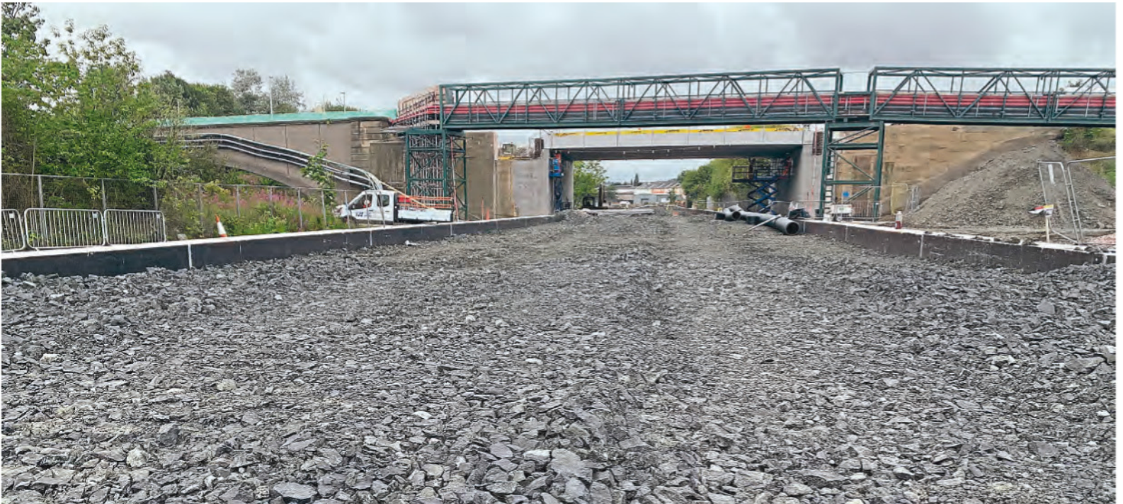
Leven platform construction. Network Rail
