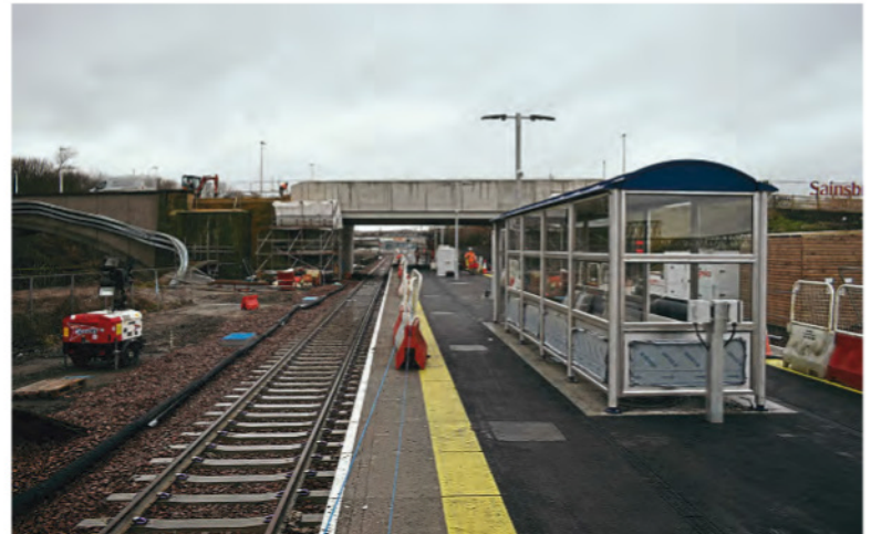
On December 15, 2023, Leven station is taking shape, with a shelter constructed and lights being erected. Richard Clinnick
