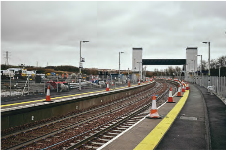
Cameron Bridge station on December 15, 2023, looking towards Leven. Richard Clinnick
